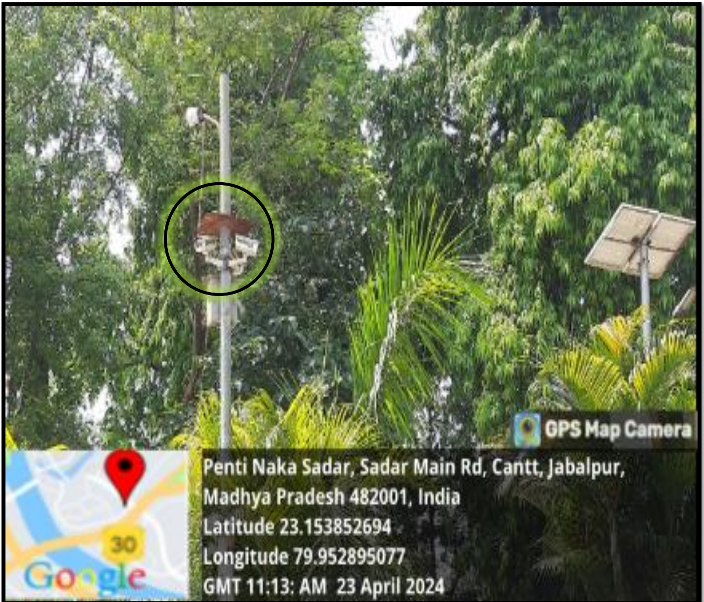
Parking & Canteen Area
